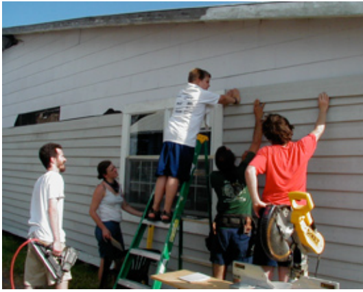
Re-siding a home in Duloc, Louisiana.
